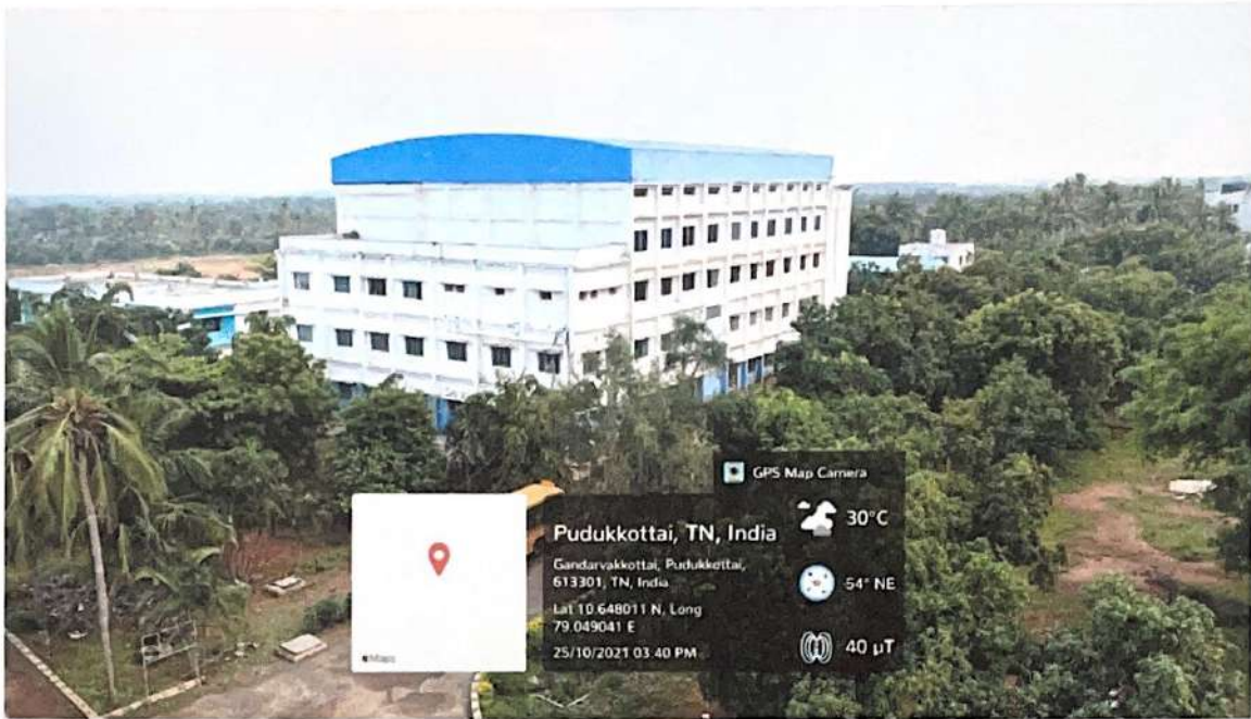
Block III ( Mechanical Block)
